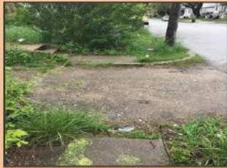
Existing Conditions: Oakley Avenue
